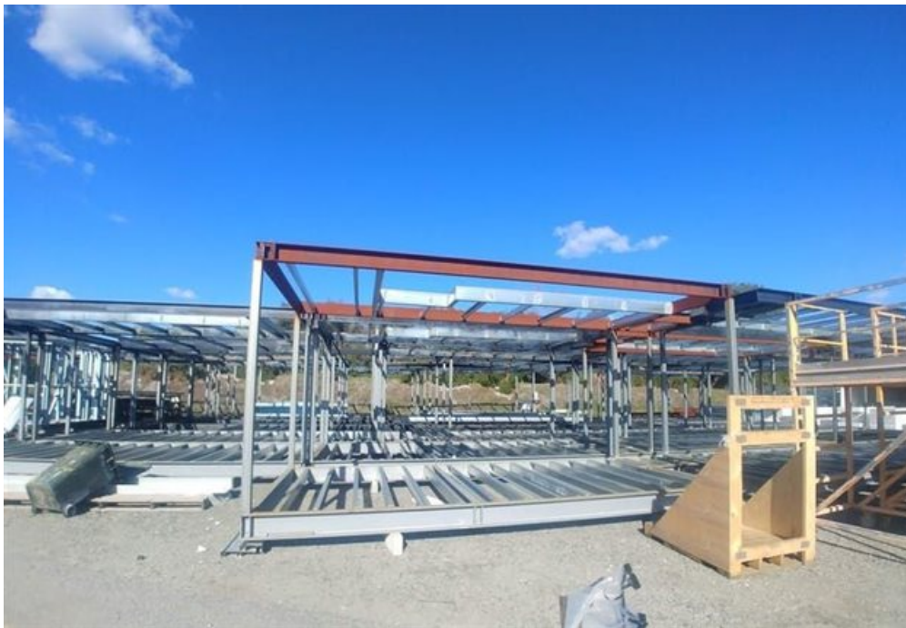
The reuse of steel frames for building saves costs and reduces resource consumption and emissions. Author provided
