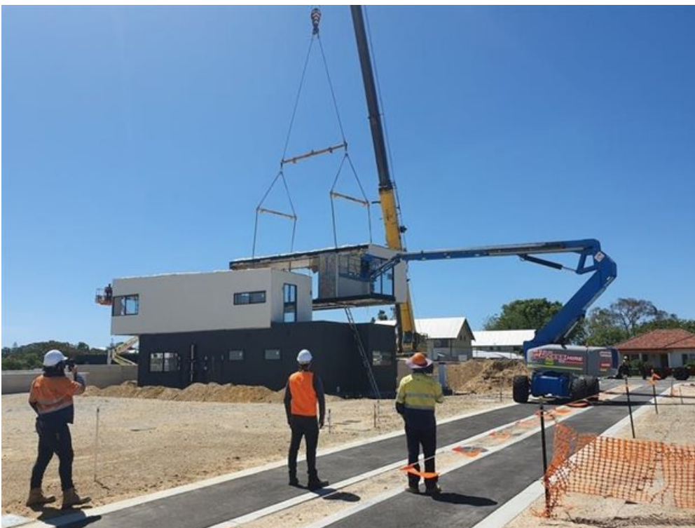
The building's eight modules were built off-site and then rapidly put together on site. Author provided
