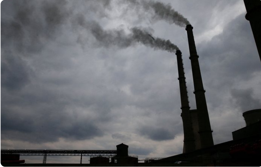
Hwange Power Station in Hwange, Zimbabwe. Source: Reuters/Phillimon Bulawayo
