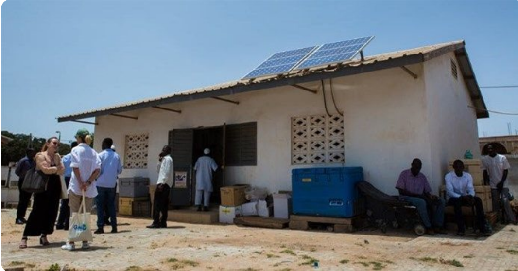
Solar energy is an invaluable resource in rural areas like this facility in Gambia. Gavi/2018/Guido Dingemans
