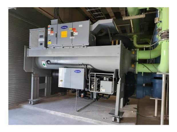
To complement the installation and serve as a backup in the event of possible future water restrictions, two existing Carrier Air Cooled Scroll Chillers from the M&M Building were repositioned. The final plant will consist of 2x 19DV and 3x air cooled chillers providing a total of 6,000kW cooling capacity.
