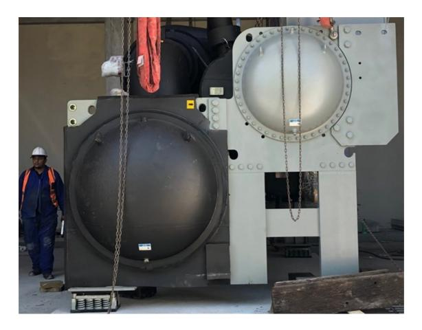
A comparative analysis of various competitive brands and load conditions revealed that the new Carrier 19DV water-cooled, variable-speed centrifugal chiller is the most suitable for the application. Here are some numbers for those interested:
